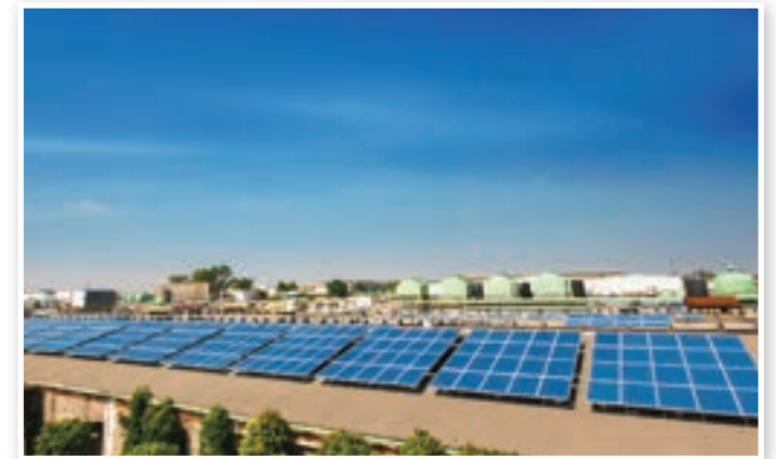
Solar panels at a shallower angle than you would see in the UK because these are closer to the equator than here
