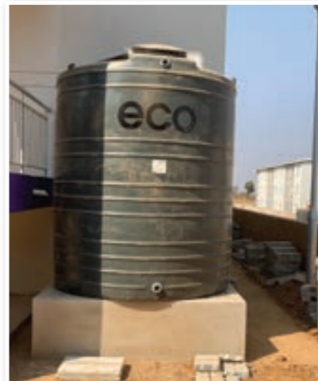
Rainwater harvesting storage at a green social housing development in South Africa
