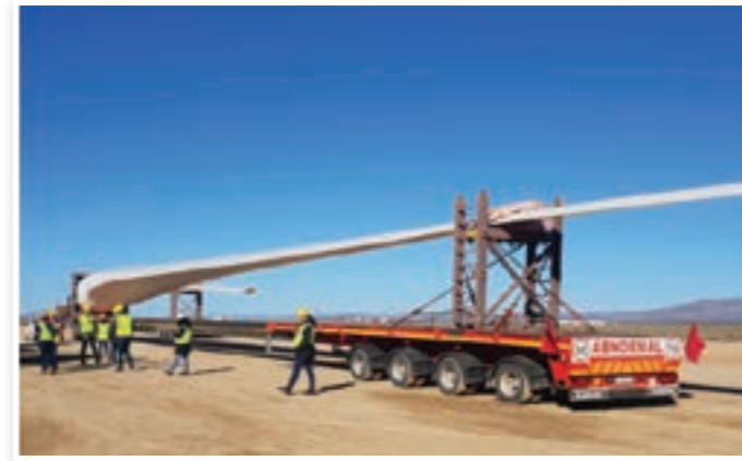
Wind turbine construction in South Africa
