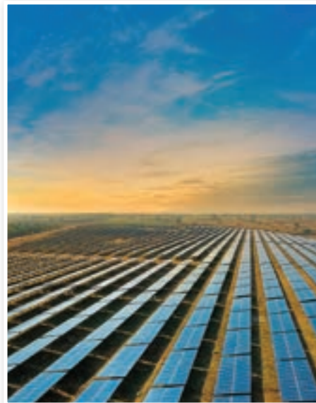
Solar Farm in India
