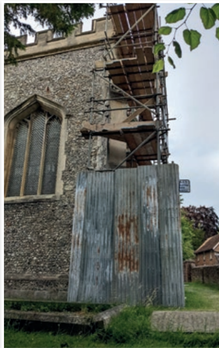
Scaffolding erected to facilitate inspections and repairs of stonework
