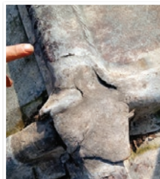
Photos of the lead roof to the turret which is in poor condition, split in places and causing leaks
