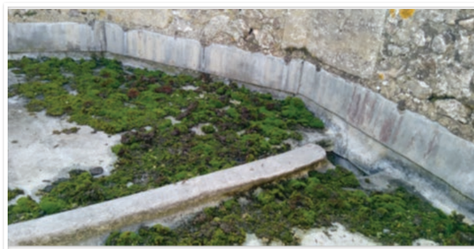
Photos of the lead roof to the turret which is in poor condition, split in places and causing leaks
