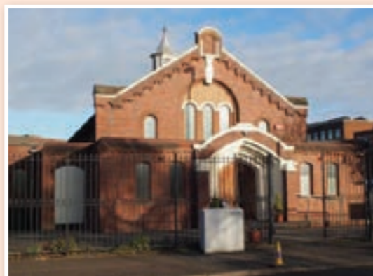
George Road Baptist Church, Birmingham
